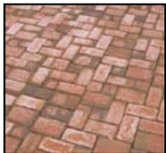
Efflorescence can be removed with cleaners specifically made for concrete pavers. Use care when applying them because many contain detergents and diluted acid. Contact your paver supplier for further information on efflorescence cleaners.
